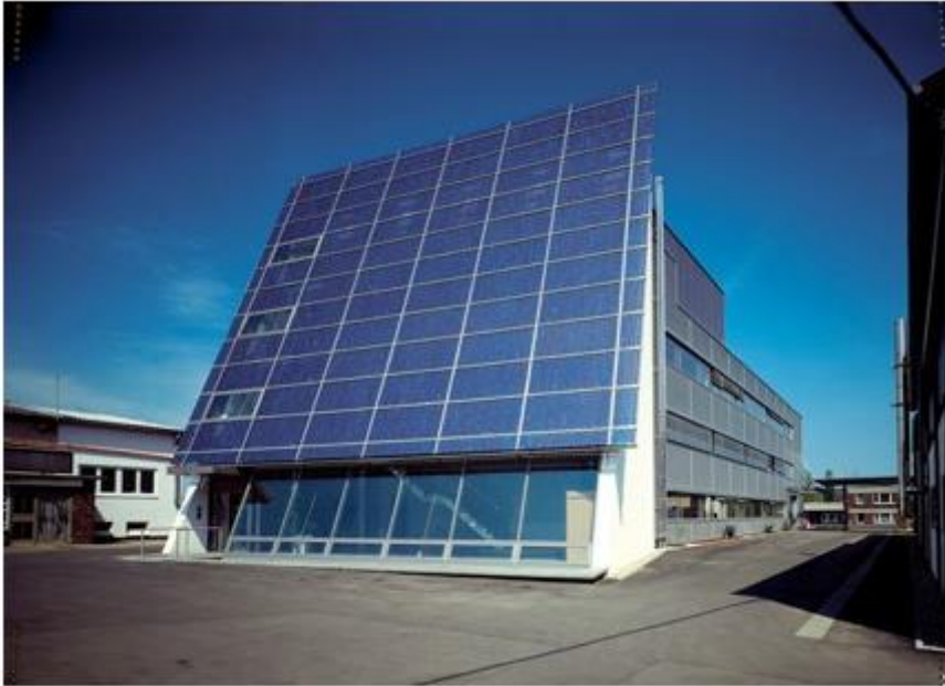
Figure: PV plant on the façade of an industrial building, source: https://www.solar mango.com/dictionary/bipv
