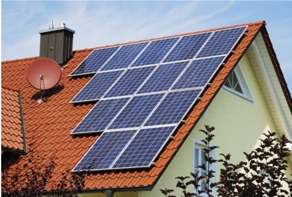
Figure: Mounting PV panels on shingle roofs,
