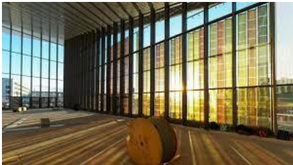
Figure: Installation featuring dye-sensitized solar cells at the Swiss Tech convention center Image: EPFL/Alain Herzog
