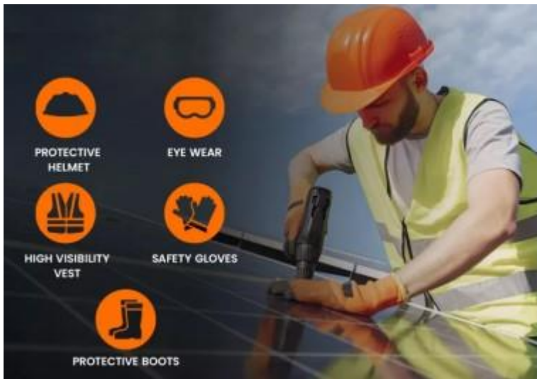
Figure: The installer and his personal protective equipment.
