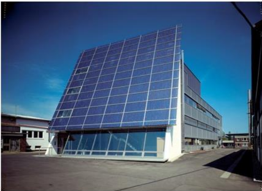
Figure: PV plant on the façade of an industrial building,
