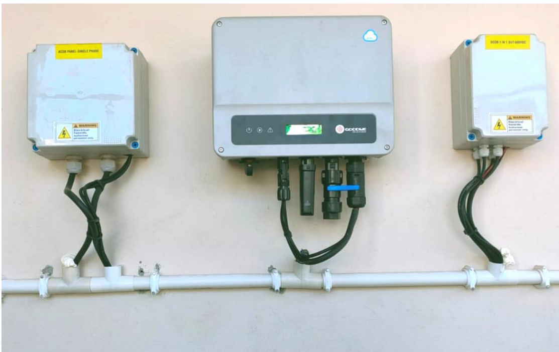
Figure: Cables in PVC or HDPE conduits provide protection. says a great influence on the overall aesthetics of the installation, source: https://www.solarsquare.in/blog/how-to-install-solar-panels/
