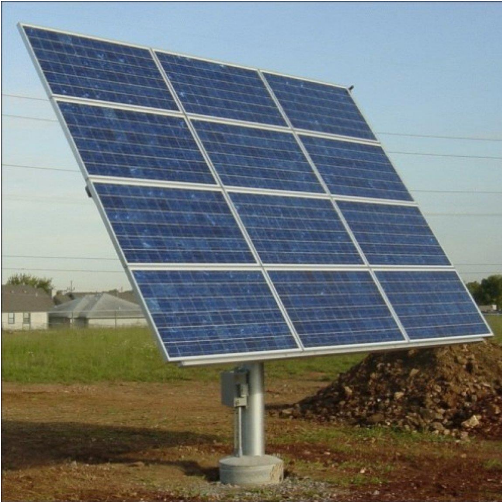
Figure: A PV tracker system , source: https://www.greentechrenewables.com/article/pros-and-cons-solar-tracking
