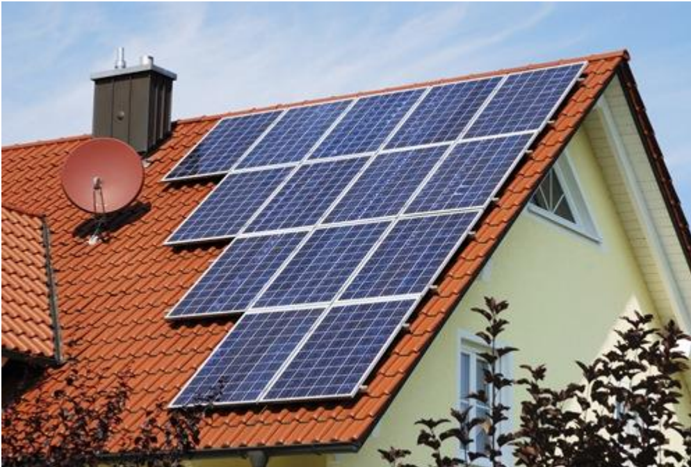
Figure: Mounting PV panels on shingle roofs,
